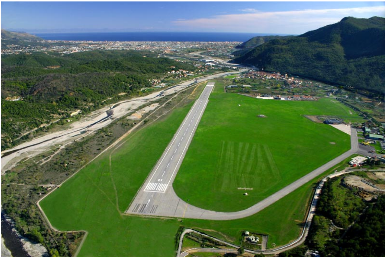
Figure 3 - Airport View from West (RWY 09)
