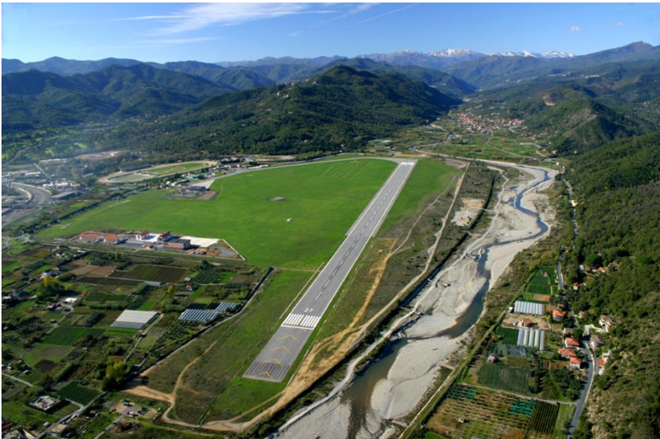
Figure 2 - Airport View from East (RWY 27)
